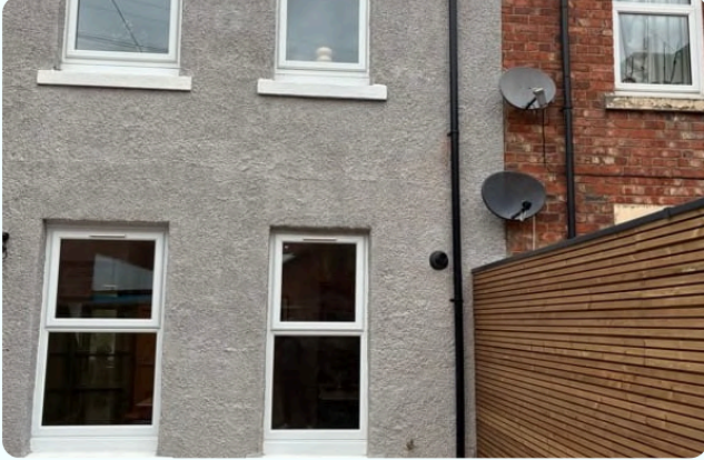
Render in good condition
