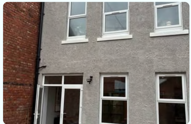
Render in good condition
