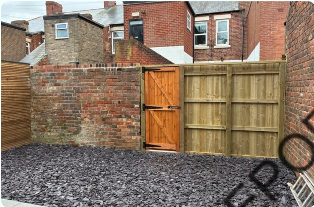
Fencing and paving well maintained
