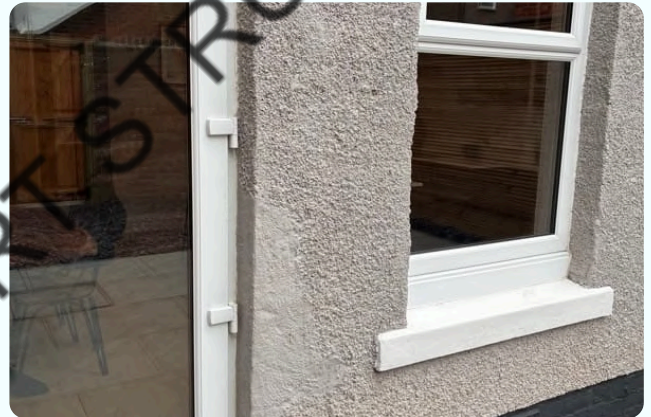
Render in good condition
