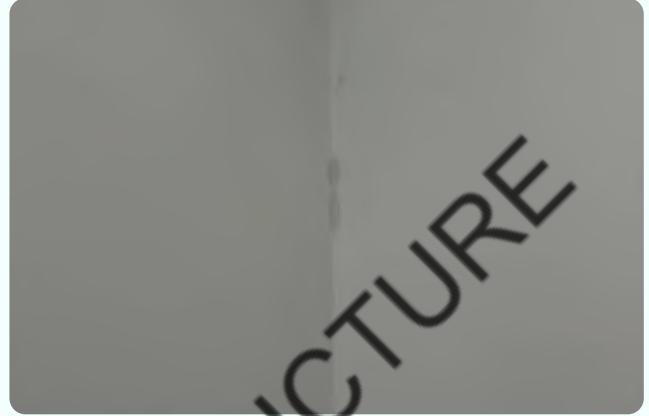
Visible damp patches on wall
